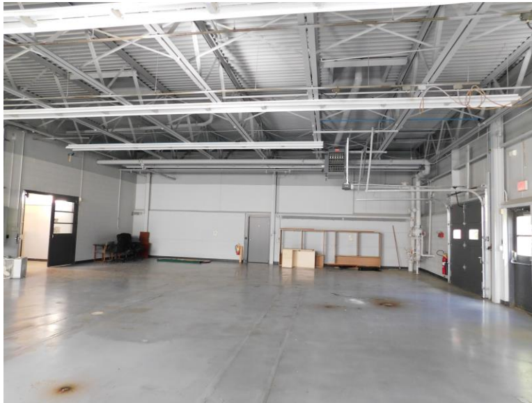
Figure 2: T12 Fixtures within the Facility
