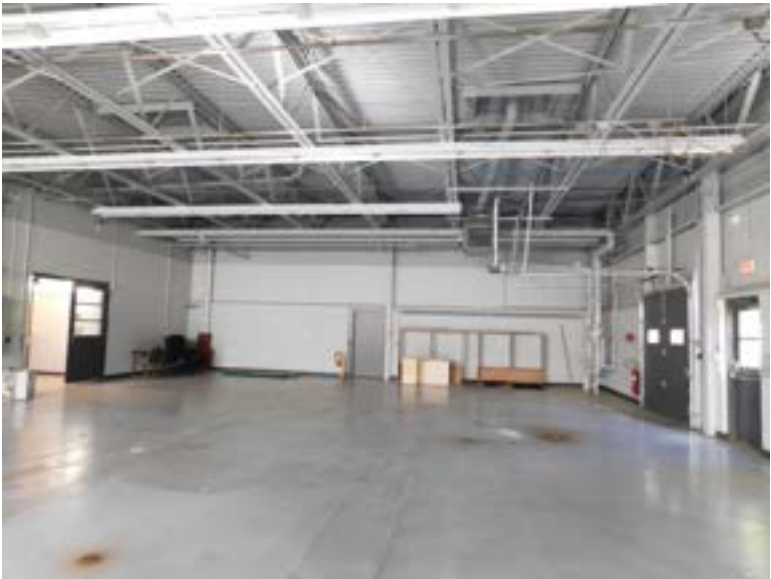
Figure 2: T12 Fixtures within the Facility
